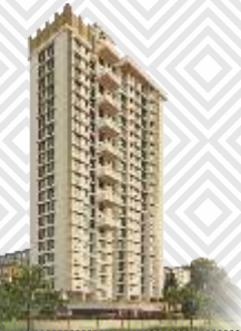
Kabra Garnet Malad (W) ONGOING
