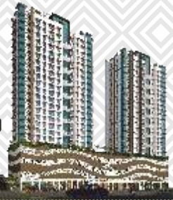
Kabra Metro One Versova COMPLETED
