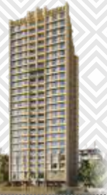
Kabra Tiara Goregaon (E) ONGOING
